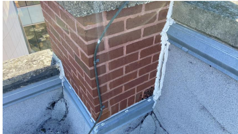
Figs. 12 and 13 – areas of sealant repair at various wall-roof intersections.
