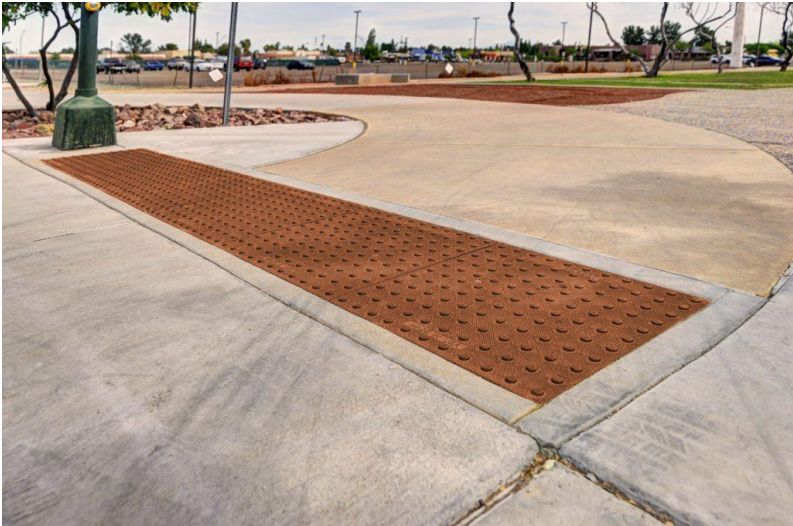
Fig. 4- Example of detectable tactile warning surface at locations where pedestrians cross paths of vehicular traffic.
