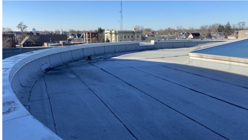
Fig. 18 - modified bitumen roofing system at building rotunda.
