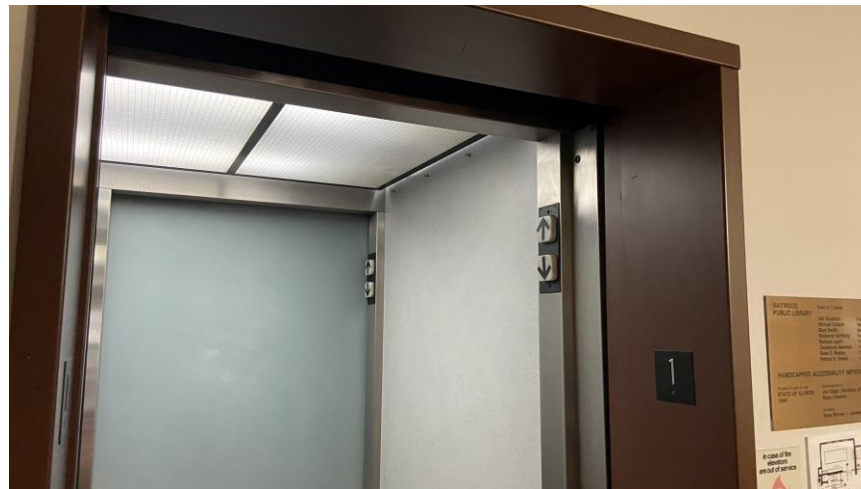
Fig. 6- Elevator door and cab at Carnegie portion of building
